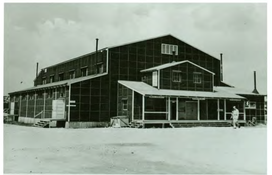
Recreation Hall - Building # T-1275 West Side of Arlington Drive between 12th & 13th Streets
